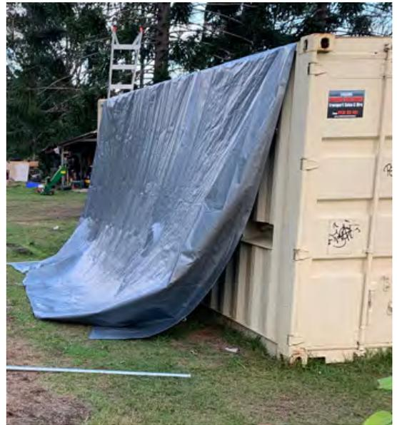
Marking out the pole position. With a person at each corner, feed the pole tips through the corner rings and stand the poles upright. While holding the poles upright, you both walk away from each other as well as the container, until the tarp is tight. Mark the pole position on the ground. Don't worry about the middle pole for now.
