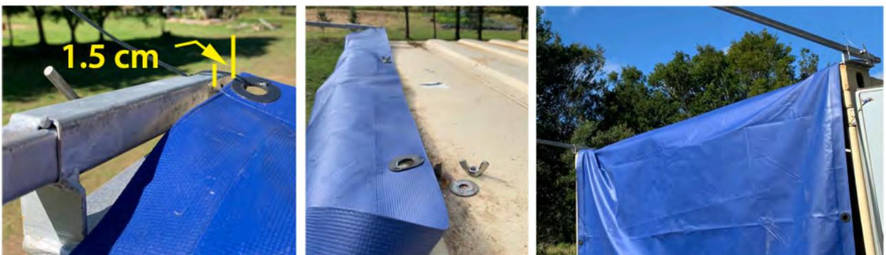
5. Take hold of one of the tarpaulin corners and hold it next to the hole in the square pole over either corner of the container (see yellow arrow above). The long side of the tarp needs to end up over the container and the short sides along the poles. Fix the corner with a cable tie, leaving 1.5 cm between the tarp's edge and the pole. The cable ties are supplied.
